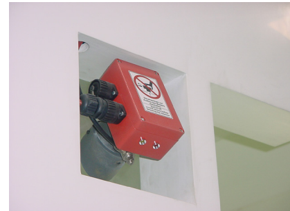
Fire detection sensor shown in situ on a ColorMax 3 fast colour change booth.
